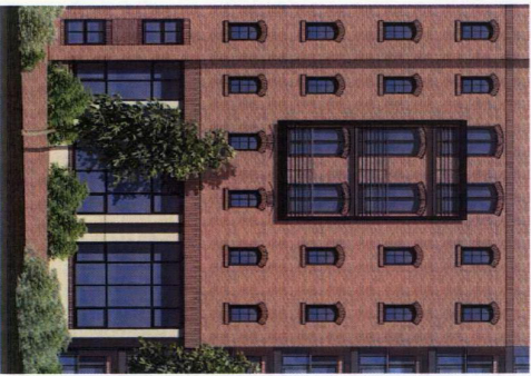
Large glazed infill panels at ground floor level with projecting balconies above
